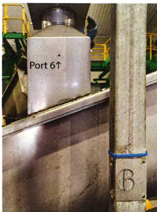
24-102: New Vacuum Port 6 (existing)
